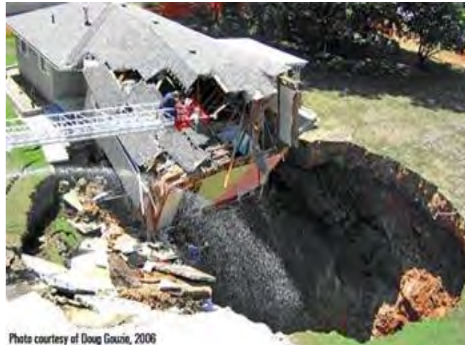
Figure D-11. Sinkhole Collapse of House
