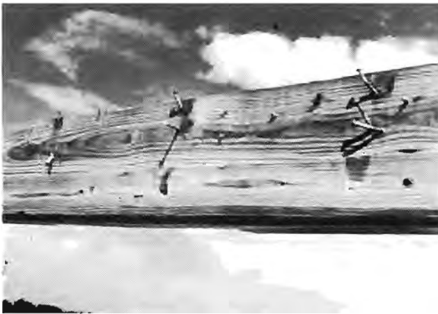
Figure 4.26. Toe Nailing Provides Limited Pull-Out Resistance
