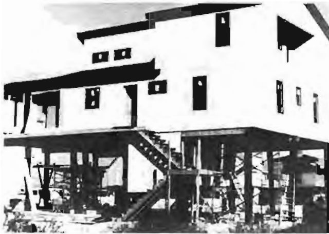
Figure 4.14. Pile Foundations
