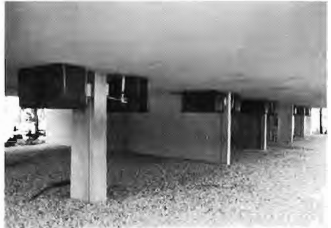
Figure 4.49. Elevated Condenser Units
