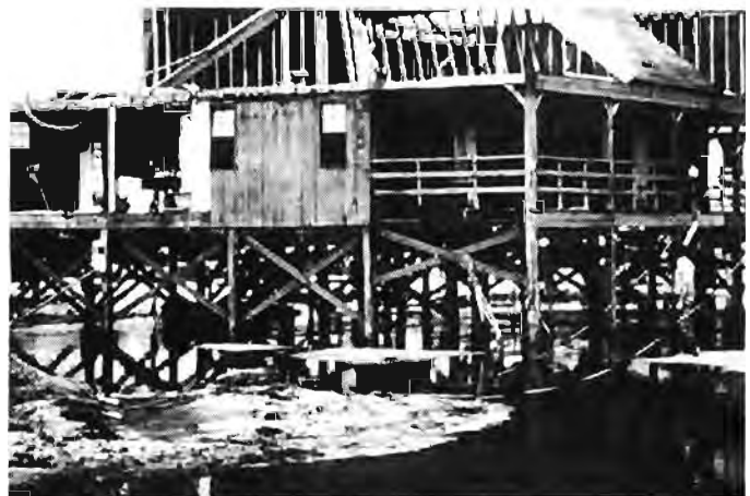
Figure 4.23. Diagonal Bracing
