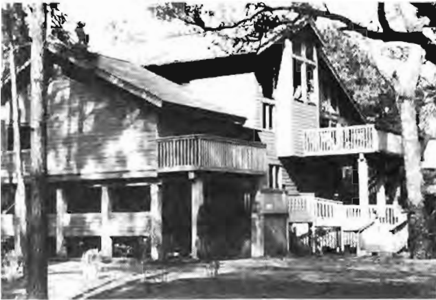
Figure 4.3. Elevation by Posts
