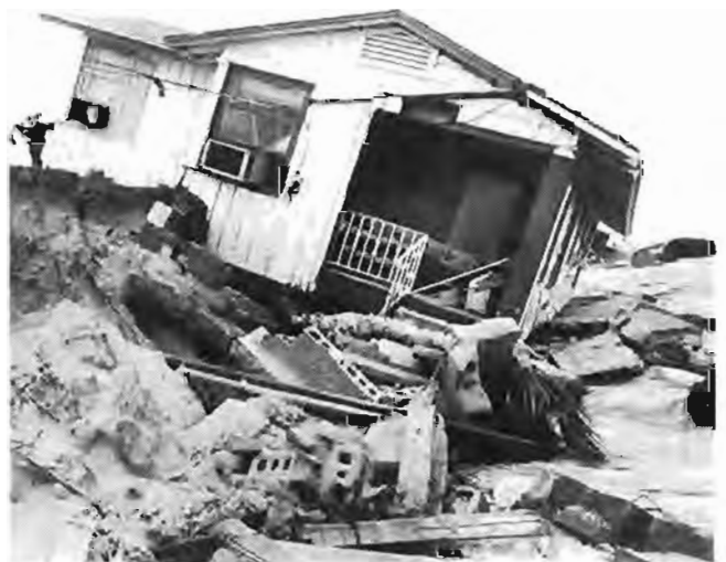
Figure 2.3. Erosion Caused This Foundation to Collapse.
