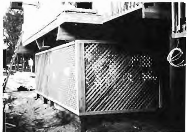
Figure 4.54. Breakaway Walls
