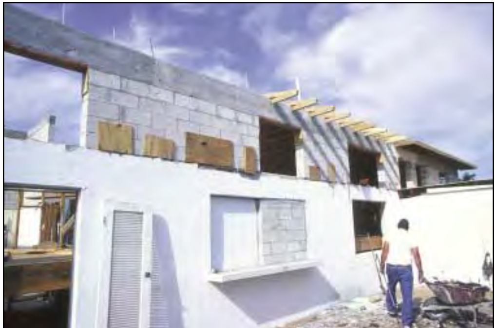
Figure 67 The extended first-story walls.
