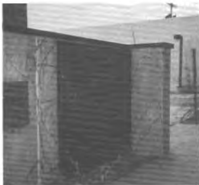
Small courtyard area is protected by combination of precast concrete wall and flood shield at door opening.
