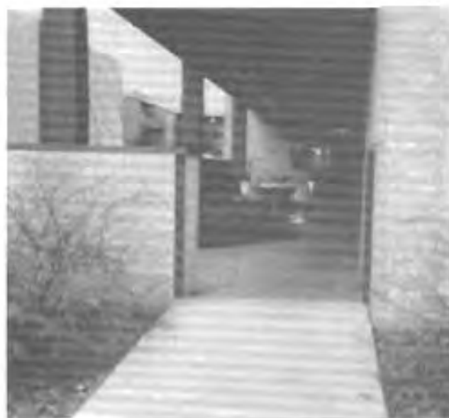
Flood shield in storage position adjacent to opening it is designed to protect.
