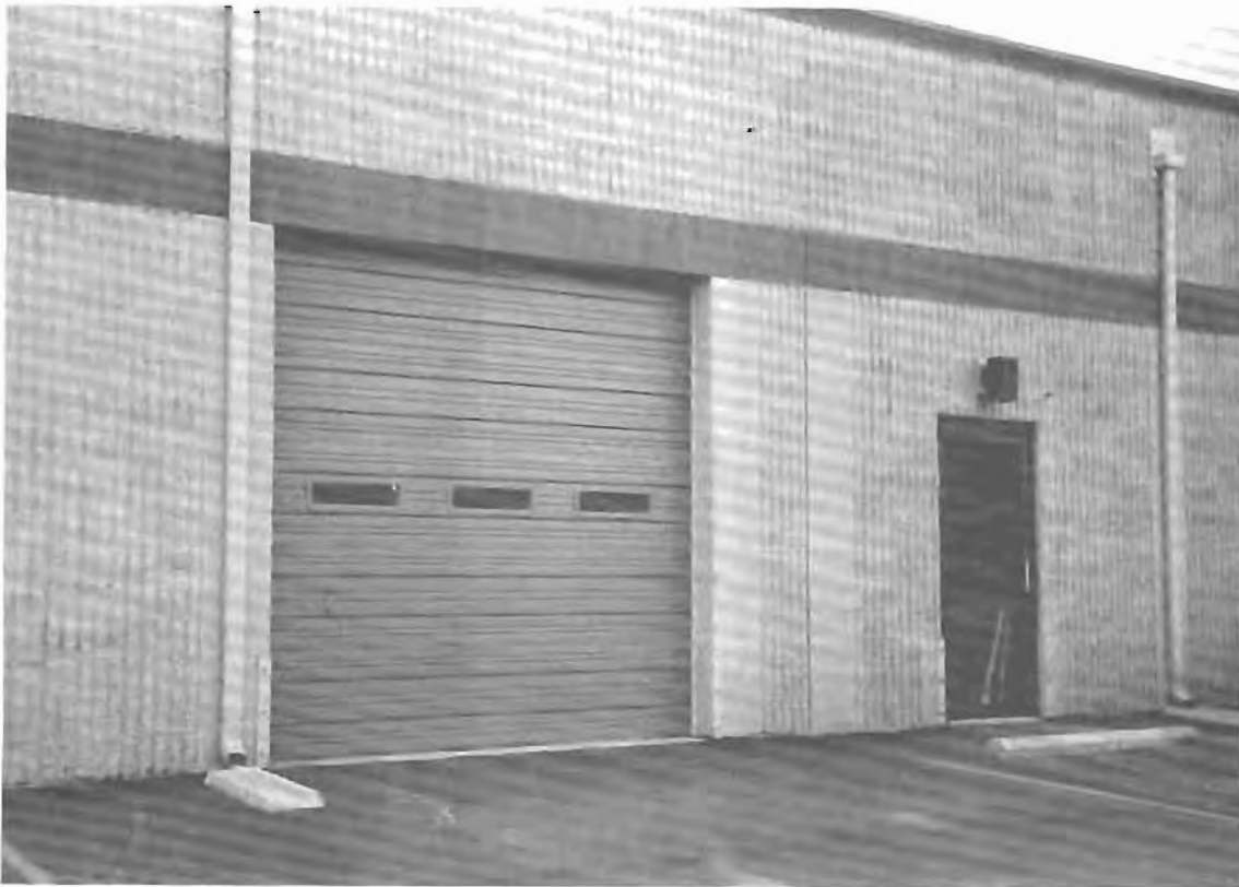
Floodproofing requires installation of 18 flood shields to protect 8 vehicular entrances and 10 personnel doors.
