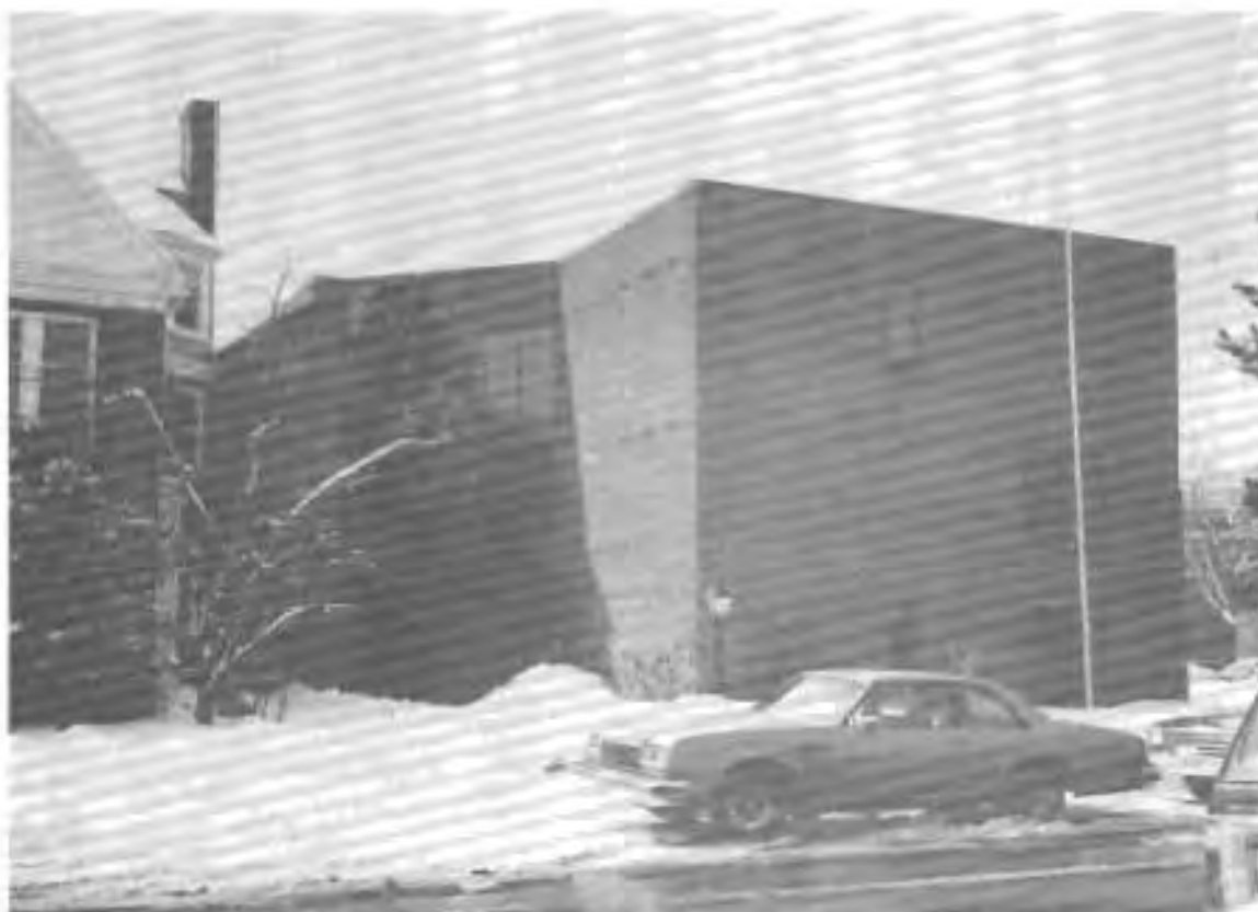
Structure has been elevated 7 feet above the base flood level in recognition of potential damage from floods that exceed the regulatory flood level.
