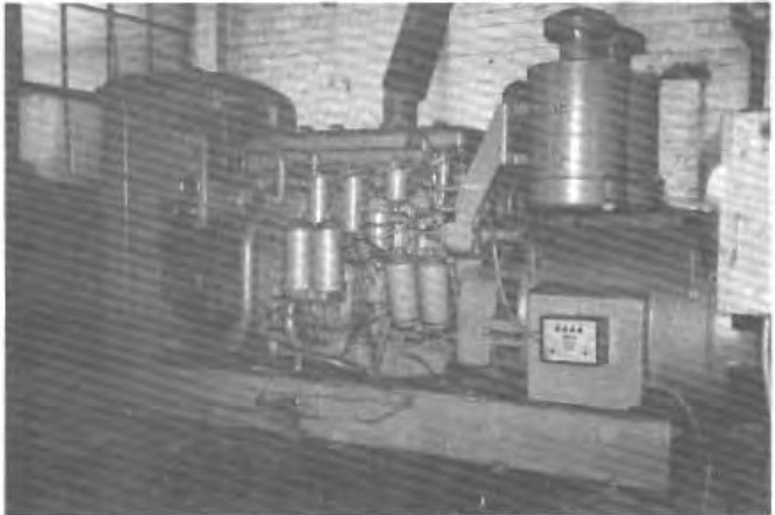
Diesel pump which can be used to dewater seepage within the plant and from a below grade collector system on the perimeter of the plant that is designed to reduce uplift forces on the floor system.
