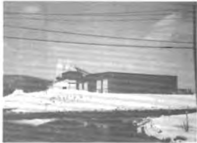
Garage structure elevated on earth fill.
