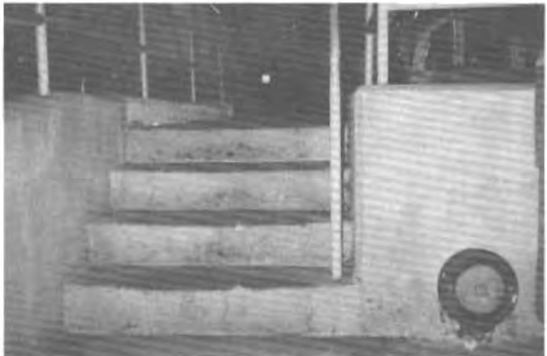
Newly constructed computerized rolling mill area has been elevated above the base flood elevation.
