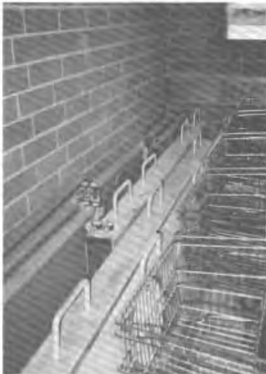
Stored flood shields (Note pneumatic seal valves).
