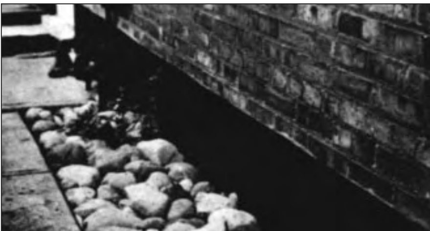
Figure 7-7 a 12-inch-high asphalt coating was added to this brick wall.
