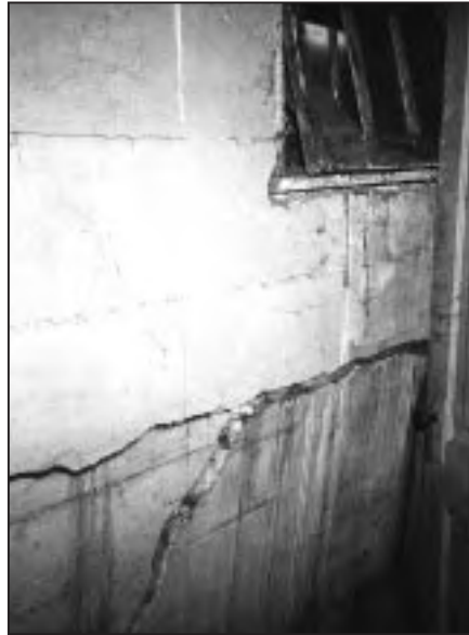
Figure 2-8 The walls of this basement in North Dakota failed because of the pressure exerted by water and saturated soil.
