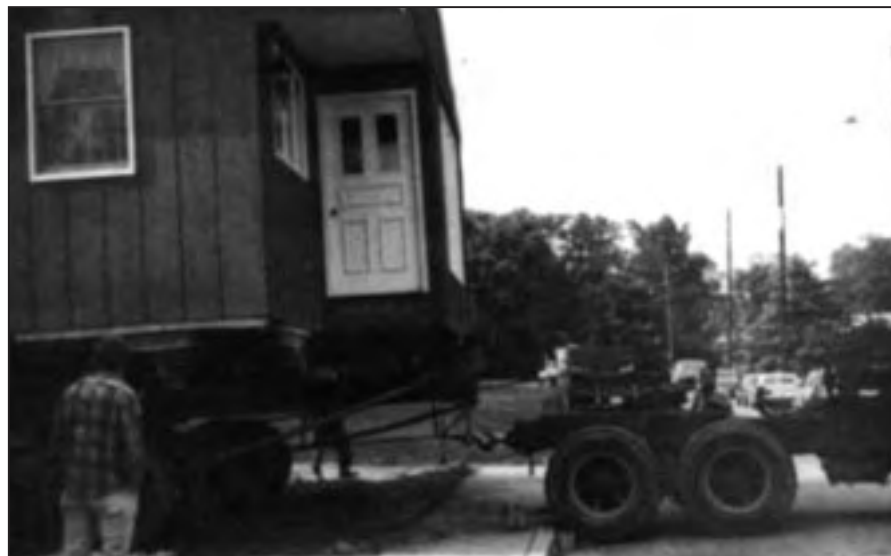
Figure 7-3 The journey to the new site begins.
