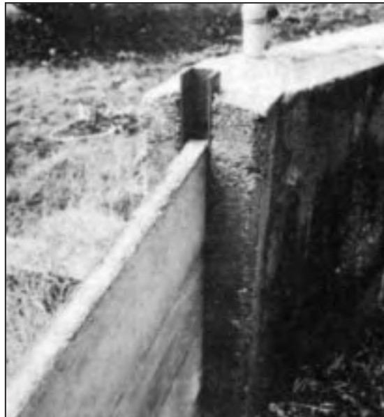
Figure 7-16 Slide-in closure panel.
