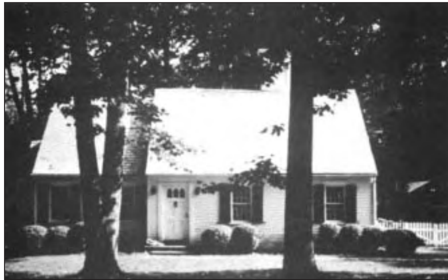
Figure 2-1 This house near Atlanta was flooded several times. During the largest flood, the water reached as high as 2 feet above the first floor.
