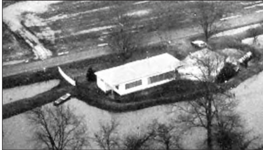
Figure 3-11 House protected by levee, which holds back the flood waters shown in the lower half of the photograph. Note that the levee ties in to high ground created by the road embankment.
