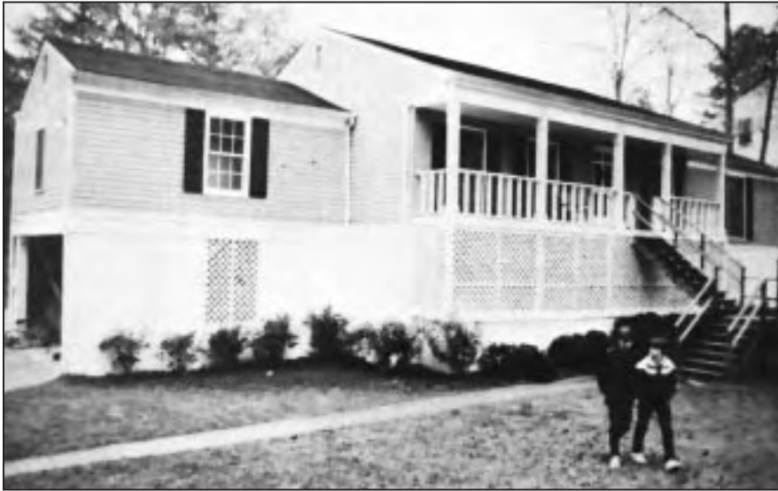
Figure 5-2 This house in Atlanta, Georgia, was elevated one full story. The garage and storage area are at the house's original elevation.
