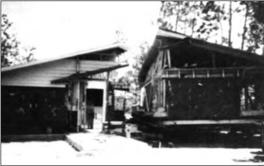
Figure 7-1 When a house is too large to be moved in one piece, it must be cut into sections that can be moved separately and then reassembled at the new site.
