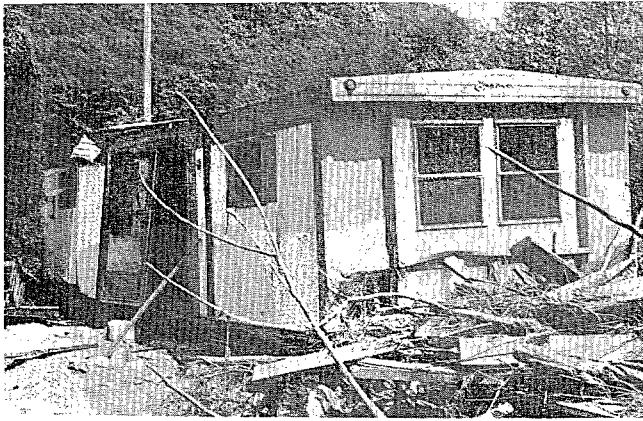
Figure 2.4 Damage From Debris
