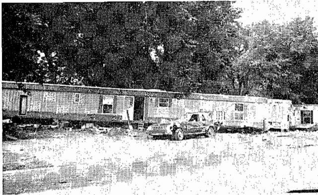
Figure 1.22 Flash Flood Damage
