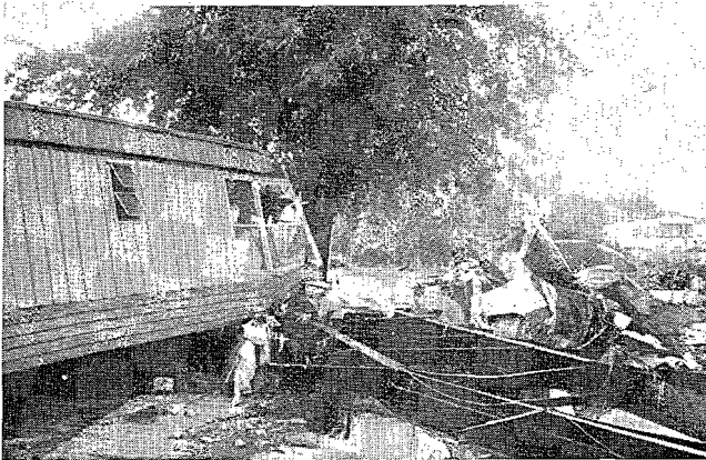
Figure 1.15 Movement From Foundation
