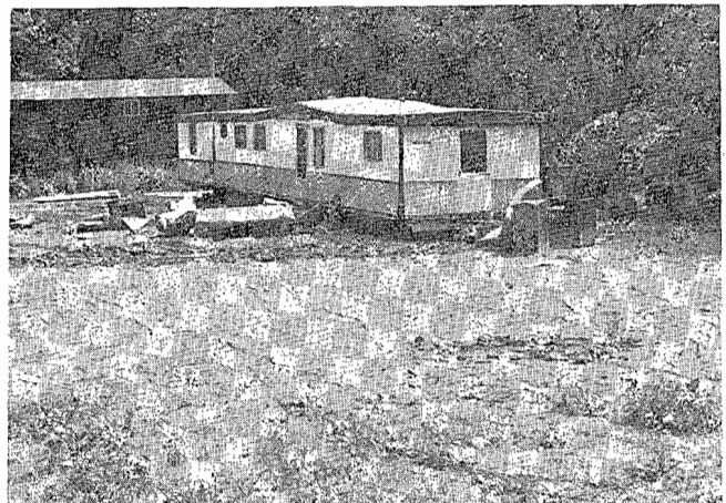
Figure 1.24 Shallow Flooding Damage
