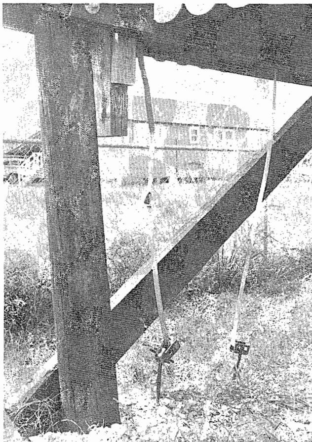
Figure 3.23 Knee Bracing
