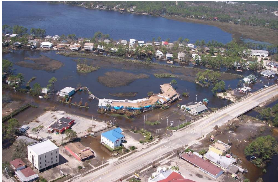
Figure 5.4 – Hurricane Ivan Damage, Gulf Shores, AL
