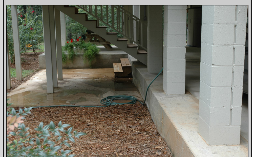
A new 3-foot concrete slab foundation was poured before elevating this house on cinder block piers to mitigate against flooding.
