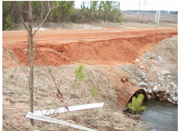
Photo 4: Example of fill placement without BMPs.
