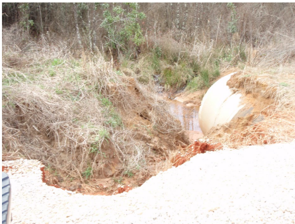
Photo 5: Lack of adequate outlet protection.
