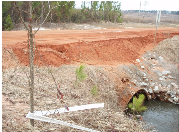
Photo 4: Example of fill placement without BMPs.
