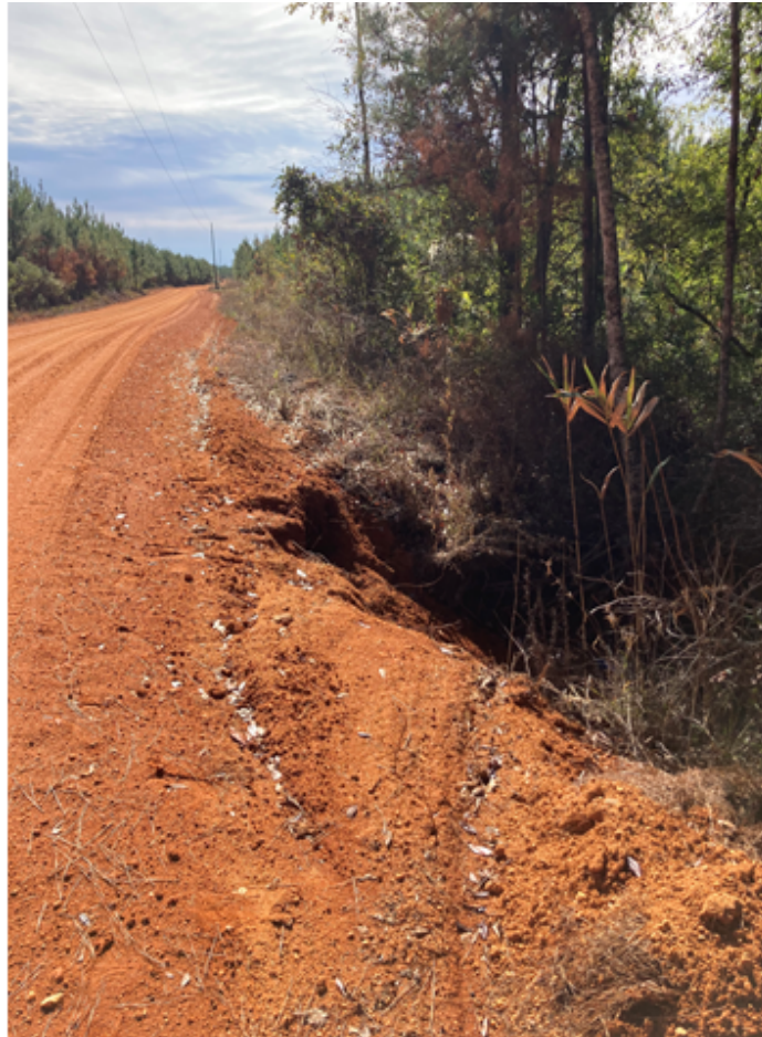
Erosion at Culvert to Creek
