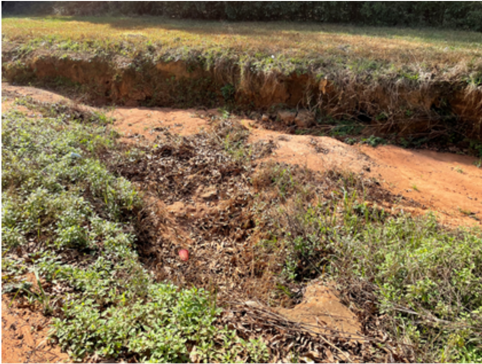
Roadside Right-of-Way Erosion-Flows to Channel
