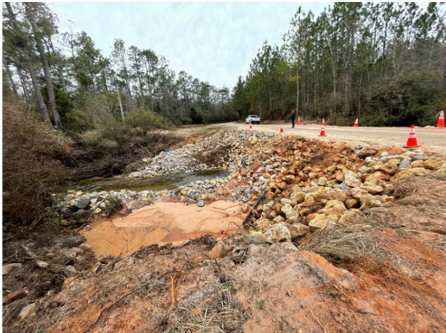
Erosion Noted at Reedy Creek Culvert
