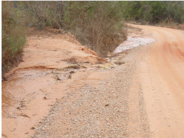
Photo 3: Example of failed “turn-out”.
