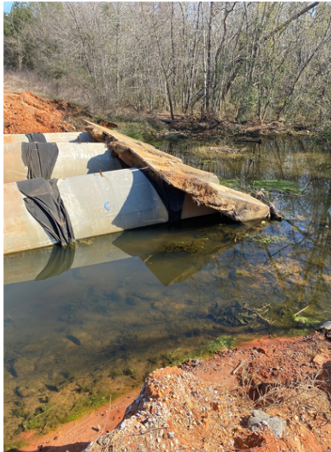
Damage of Culvert System During Hurricane Sally
