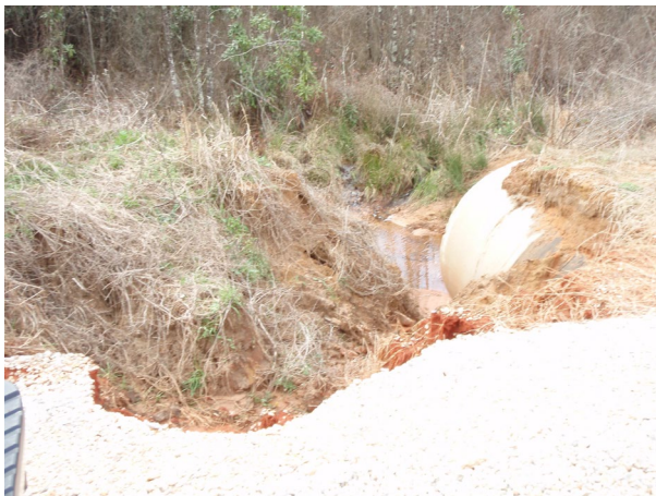
Photo 5: Lack of adequate outlet protection.
