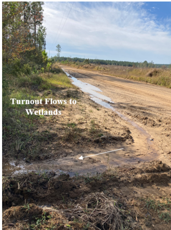
Stormwater Turnout Directed to Wetland
