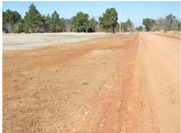
Photo 8: Typical staining associated with turbid runoff.
