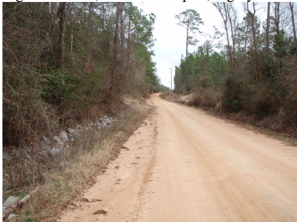
Photo 1: Example of previous ditch line treatment.
