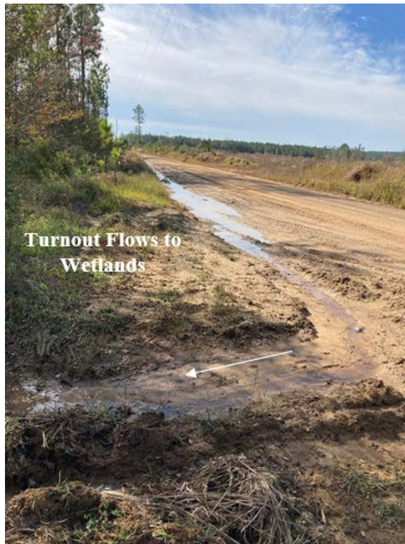
Stormwater Turnout Directed to Wetland
