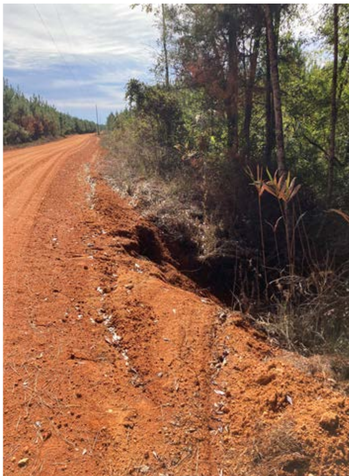
Erosion at Culvert to Creek
