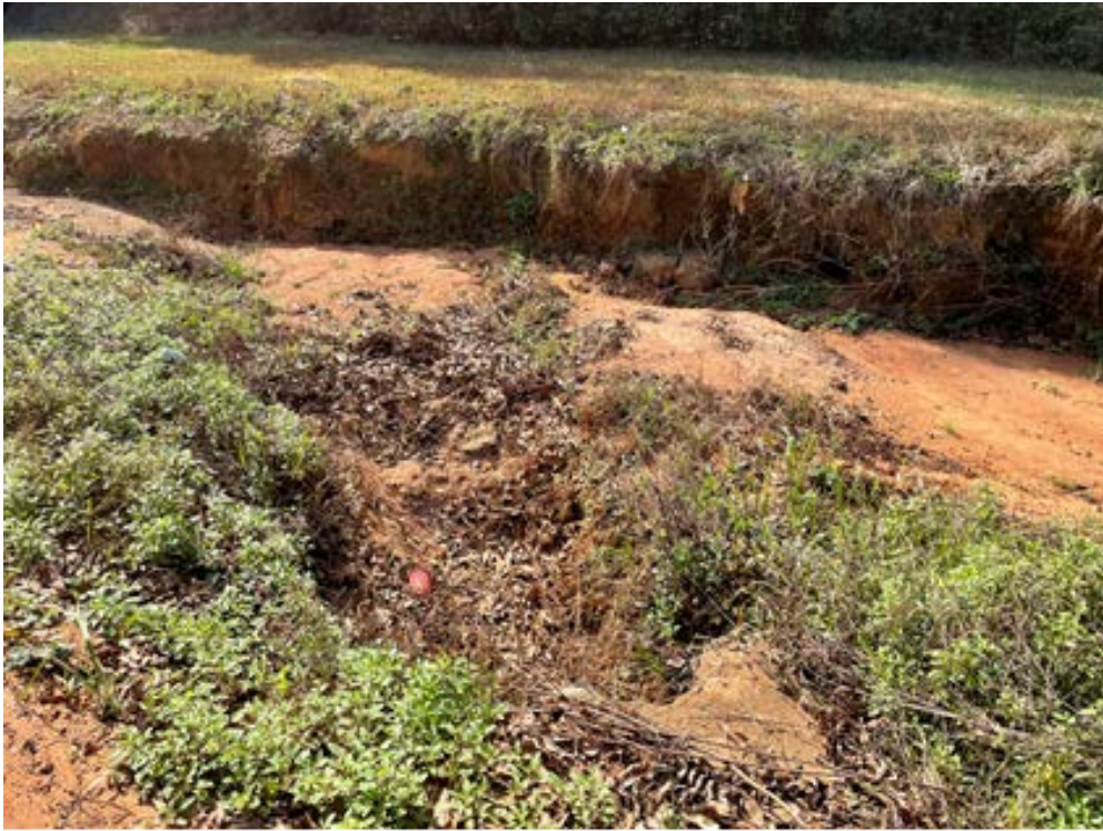
Roadside Right-of-Way Erosion-Flows to Channel
