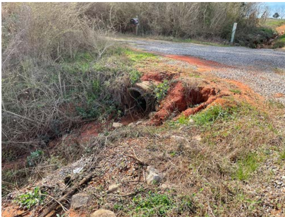
Erosion Near Road Culvert Flows to Wetlands and Stream
