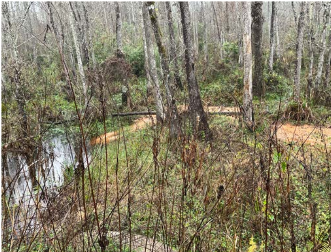
Sediment in Wetlands at Road Culvert
