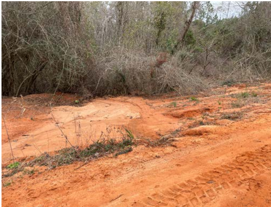
Road Eroding into Wetland Bottom
