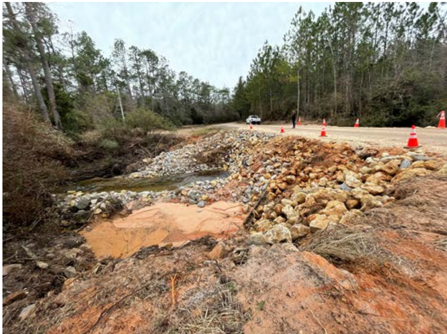
Erosion Noted at Reedy Creek Culvert
