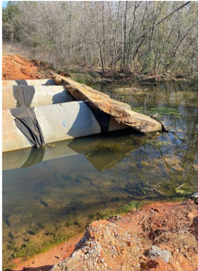
Damage of Culvert System During Hurricane Sally
