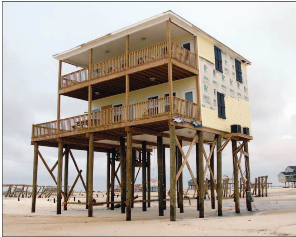
Figure 2-14. Successful example of well-elevated and embedded pile foundation tested by Hurricane Katrina. Note adjacent building failures (Dauphin Island, AL, 2005)
