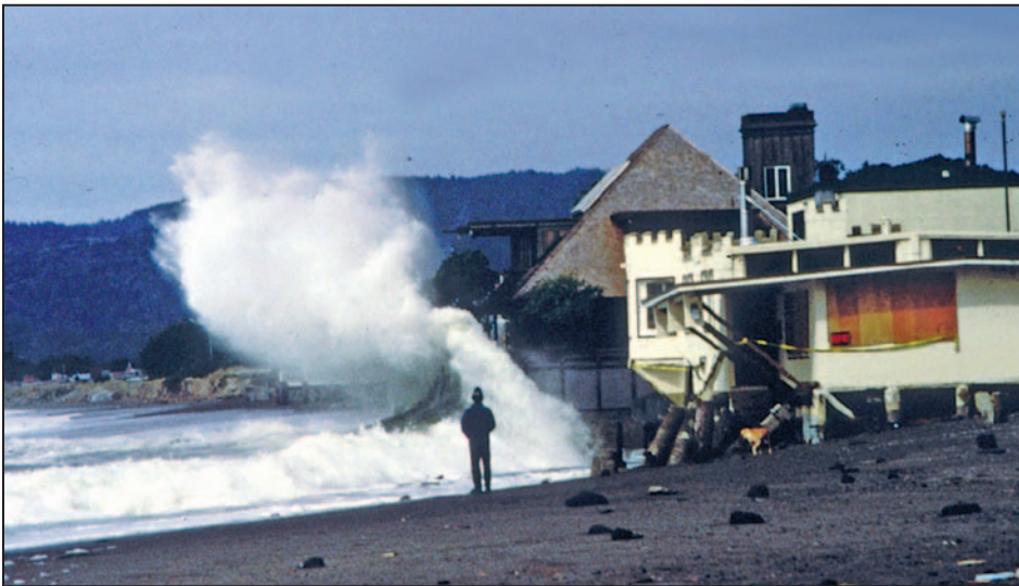
Figure 3-23. Storm waves breaking against a seawall in front of a coastal residence at Stinson Beach, CA
