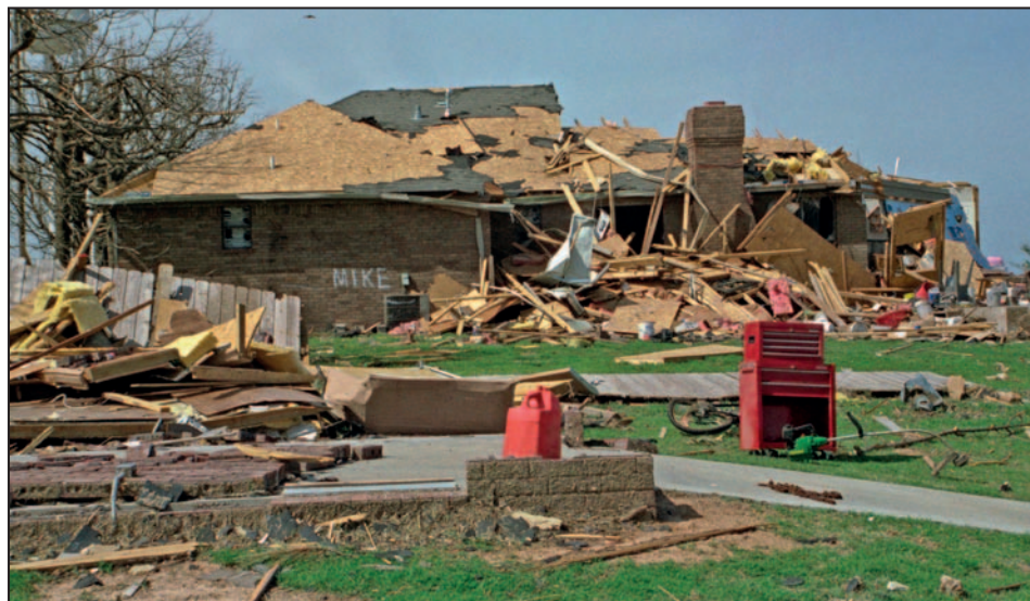
Figure 2-4. Roof structure failure due to inadequate bracing and inadequate fastening of the roof deck, Hurricane Andrew (Dade County, FL, 1992)
