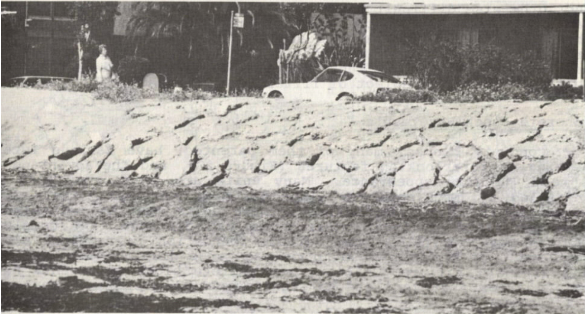
Figure 22 Concrete Rubble Revetment
