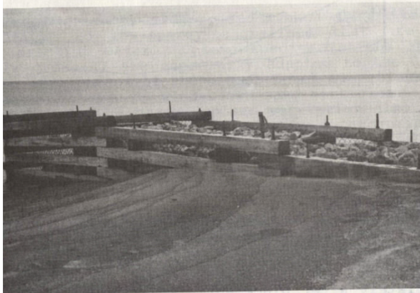
Figure 51 Timber Crib Groin
