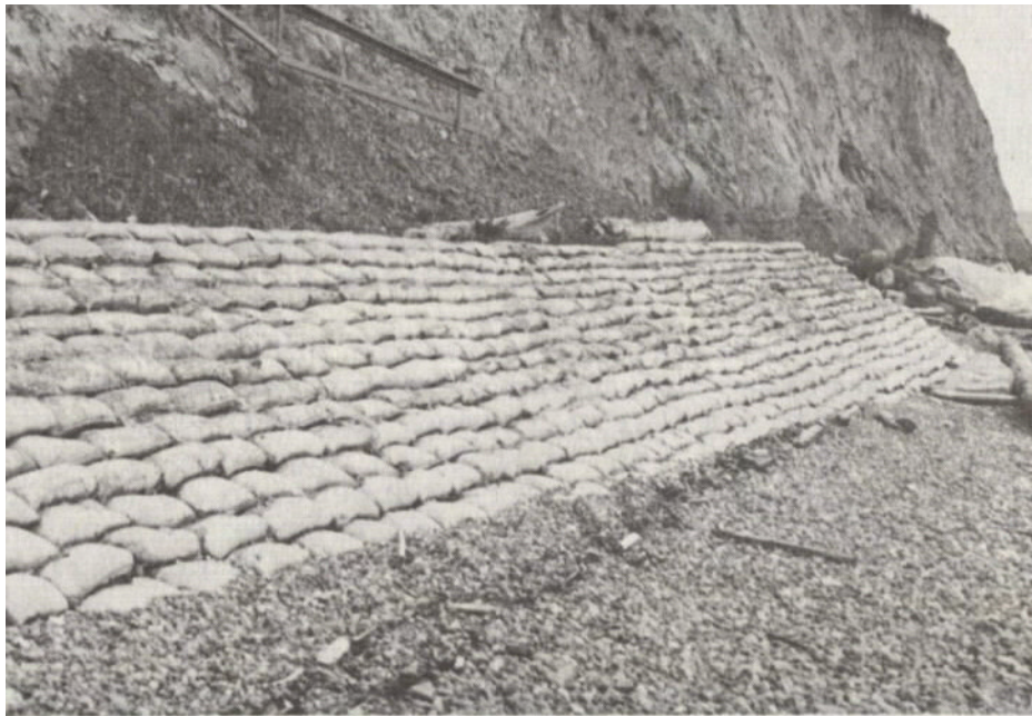
Figure 30 Stacked Bag Revetment
