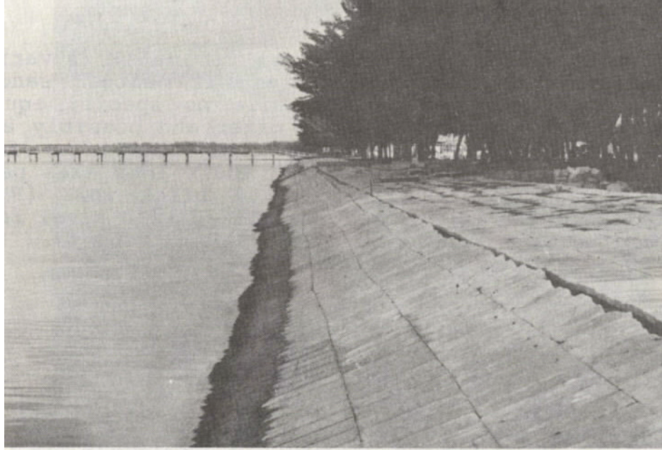
Figure 28 Lok-Gard Block Revetment
