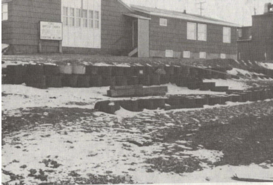
Figure 34 Steel Fuel Barrel Revetment
