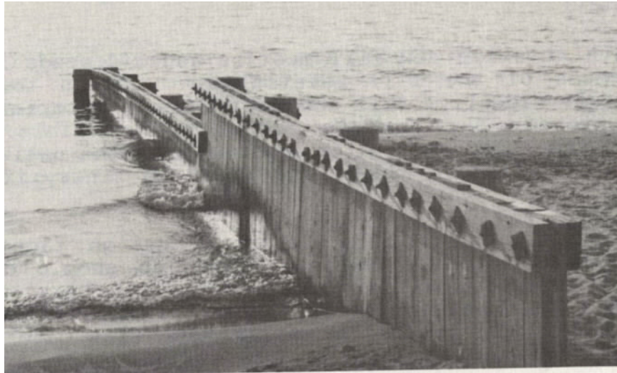
Figure 50 Timber Sheet Pile Groin
