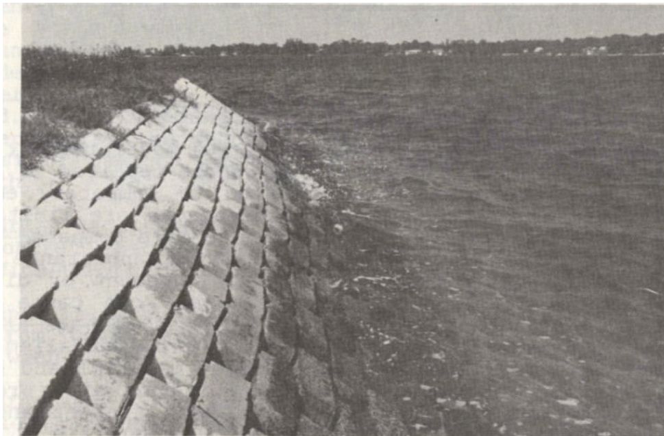
Figure 29 Terrafix Block Revetment (Photo Courtesy of Erosion Control Products, Inc.)
