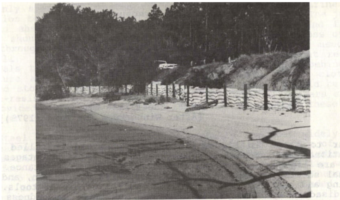
Figure 14 Hogwire Fencing and Stacked Bag Bulkhead
