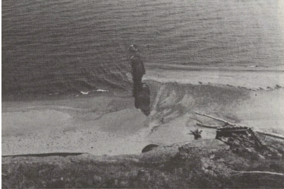
Figure 49 Longard Tube Groin
