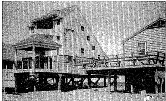
Residences are typically elevated on pressure-treated, cross-braced wood piles. One local contractor constructs over 25 residential elevation projects a year.
