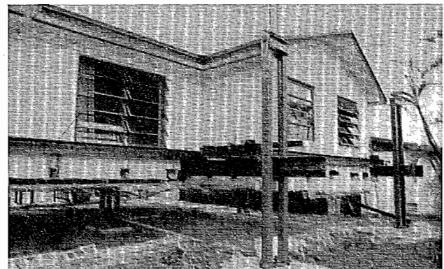
FEMA evaluated seven alternatives for elevating a typical home following Hurricane Andrew. Costs ranged from $14,400 to $36,900 for raising a home one to three feet, and from $21,400 to $41,900 for raising a home eight feet.
