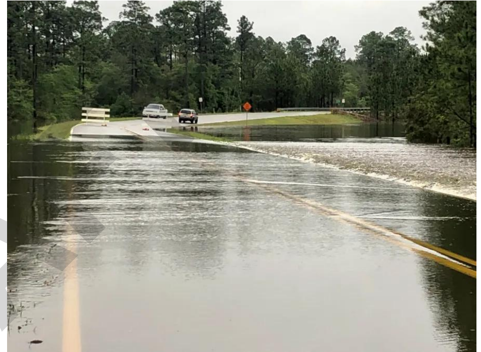
Above: Road closure in Baldwin County caused by flooding.
